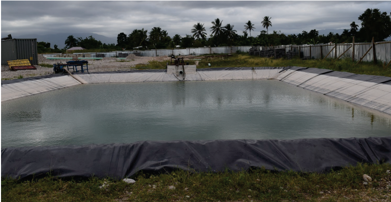
A settling pond is located near the wet vibrating screen as a source of water and to allow the washings from the sand to settle.
