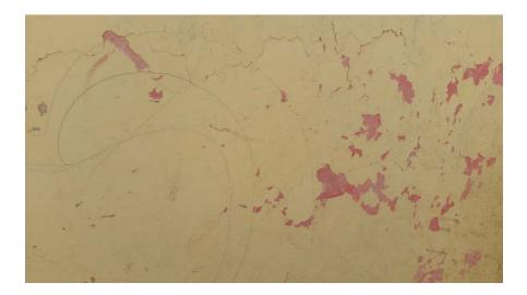
This photo shows the peeling paint on the exterior walls. This is a sign that the outer walls have a long-term moisture problem. Peeling paint was covered by paint
