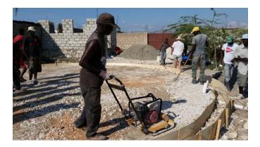
need to fill with base material way beyond the top of the inner form boards. After the compacting started, there was a lot of extra work that had been done that had to be undone.
