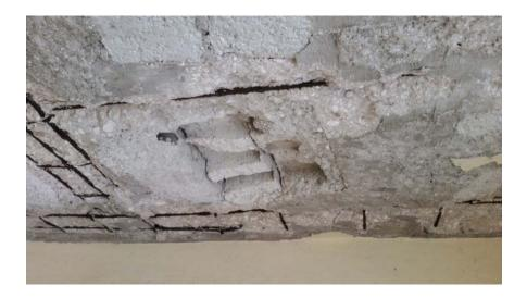
Concrete block were used as space fillers in the flat concrete roof. This is a typical construction method in Haiti. Many of the block were made with aggregate loaded with clay and were shorted on Portland cement. As a result Herb was able to remove pieces by hand and crush them by hand.
