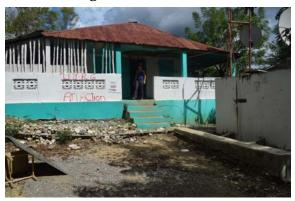
The roof was shot, and the roofing lumber was infested with termites. Apparently little rebar was used in the foundation. The left side of the building, when facing the front door, was stable. The footing for the right side of the building was about a meter lower than the footing on the left side. The right side of the building was moving downhill. There were substantial cracks in the concrete in
