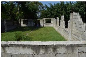
On the property is the start of a church. Footings are in and some of the walls have been installed. Some of those walls have collapsed. The footings and bond beam appear to be in good shape, but the footings need to be plastered to protect them, and soil needs to be moved to allow water to pass the structure without eroding the footings.
