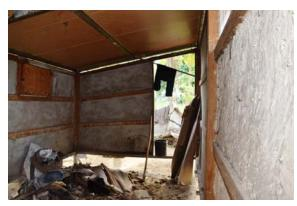
to ceiling height. Metal cross pieces at slab level and at roof level attached to the uprights. Horizontal 2x lumber was then bolted to the metal framing. The lath was nailed to the horizontal 2x lumber with 4d nails that were pounded halfway in and then bent over. This photo shows the Red Cross house that remained in the best condition.
