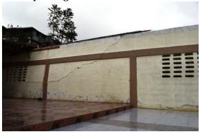
plane. It appeared that a downdraft on the trussed metal roof caused the roof trusses to exert outward pressure before failing. This cracked the wall. The small photo to the left shows one of the columns in the wall that cracked.
