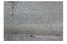
a good chance that the area below the crack has an inadequate foundation and that the foundation has been depressed a small amount.
