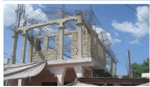
Many people have the resources to build the first story of their two- or three-story home. They leave rebar trusses sticking out so the next story can be added. Every place I have been in Haiti where concrete construction takes place, I have seen this. There are a couple of problems. The rebar trusses sticking up are exposed to the
