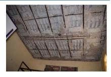
Much of ground water near the coasts of Haiti contains elevated levels chlorides. There are lakes which are at higher elevations which also have elevated levels of chlorides. If there is a chloride problem, either the steel rebar needs to be protected or a non-corrosive substitute needs to be used. Not all protection of steel rebar provides long-term protection.
