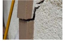
Failure to place the rebar in the proper elevation of a concrete pour also results in insufficient reinforcement. This is especially true.
