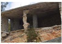
Failure to consolidate all concrete in all beams and columns is asking for premature failure.
