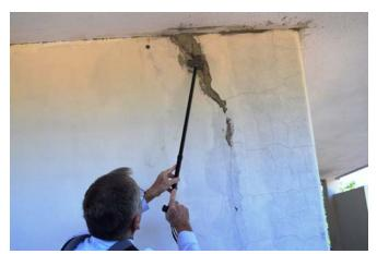
never seen these problems before. Once they saw a type of problem, their eyes were opened and they would go ahead of me to find more problems of the same type. Apparently the movement of the roof slab in relation to the support structure was the result of landing helicopters on the roof. I was informed that
