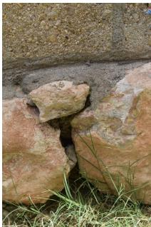
Photo was taken at the rear of the building, on the left side, and illustrates how the block wall is not tied to the column, how the block in the wall are not bonded together with mortar, but just held apart with mortar, and how the mortar between the rock of the foundation has eroded. There is also erosion on the lowest concrete block shown in the photo. In other areas of the building there was much more erosion in some of the concrete block.
