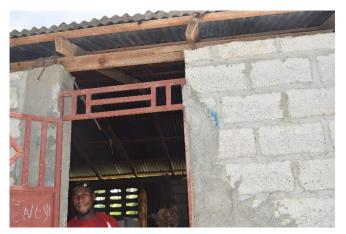
The upper portion of the same door frame. On the latch side of the door frame, repairs have been made because movement of the door frame had broken the block which were to hold it in place. There is no concrete beam above the doorway to help hold the door frame in place. A wooden beam rests on
