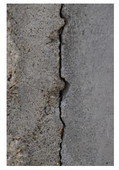
The foundation was made of fairly large rock that were mortared together. However, some of the mortar was weak and had eroded away.
