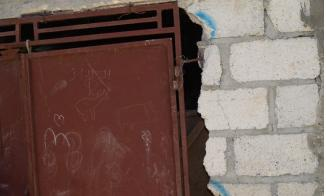
weak, and the cells were not filled with concrete, movement of the frame caused the concrete block to break. The only thing holding the door frame in place is that it is sitting on the slab, and it is nominally attached to the beam above it.
