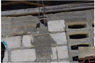
across the top of the wall. The concrete left gaps so neither the beam nor the column is effective. Further, the photo illustrates that the wooden top plate is not attached to the wall for at least one meter.
