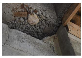
shows that the rebar truss which was to be tied through the support beam was bent over and not attached to the beam when the beam was poured.
