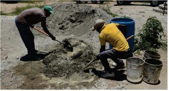
While I prefer that mortar be mixed in a mortar box using a concrete hoe, it was being mixed on the ground using shovels. This is a common way mortar is mixed in Haiti and often results in poorly mixed mortar. The crew was doing a much better job of mixing the mortar on the ground than is usually done.
