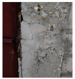
The closeup of the repair (to the left) shows the low quality of the concrete and the deterioration that has taken place since that repair was made.
