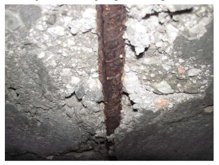
Many of the ceilings have exposed rebar and spalling concrete. Each time there is significant rainfall, more concrete spalls, and the rebar corrodes a little more. 13 Exterior stairways with unconsolidated concrete and no guard rails are common in Haiti.
