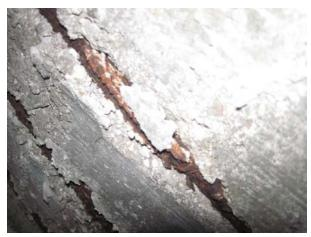
Much of the well water in lower elevations of Haiti is brackish. This brackish water is used to produce much of the concrete. The chlorides in the water attack the steel rebar and cause the rebar to corrode. As a result of the corrosion, the rebar expands, which in turn causes the concrete to crack.
