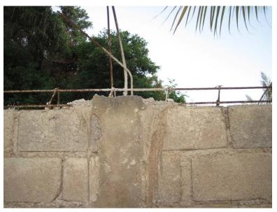
Most walls for houses and fences consist of a lightly reinforced frame with concrete block infill. Normally there are eight to twelve block between the vertical columns. The reinforced columns consist of four pieces of nominally No. 2 rebar coming out of the footing. Longer pieces are then attached: the four pieces of rebar are held into position with heavy wire placed about every meter along the
