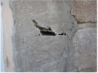
Concrete is poured in from the top and is usually rodded. However, the rodding is frequently insufficient to fill all of the voids in the column. After the concrete cures, the boards are removed. The columns are usually 10 cm or 15 cm square for fences and 15 cm square for single story houses.
