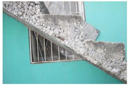
Many of the stairways have exposed rebar, spalling concrete, and unconsolidated concrete. These stairways often rely on columns to provide support. Usually, the support columns are not constructed to a higher standard than the stairway
