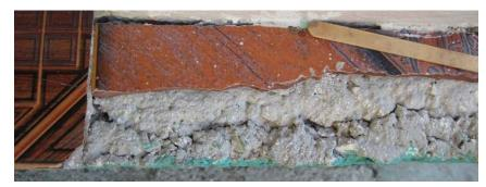
Floor tile are used to hide imperfections in concrete floors. If an adequate bedding mortar is not used, the tile are likely to break.
