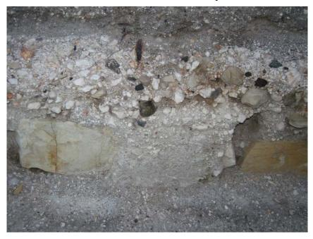
Another factor that impacts the quality of the concrete is the fine aggregate. Much of it has not been washed, and I observed some sand that contained up to 20% clay.
