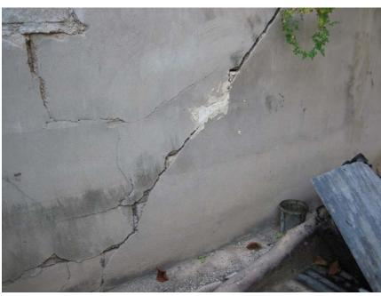
Many of the concrete walls had strong angle cracks, indicating that there was probably foundation movement.
