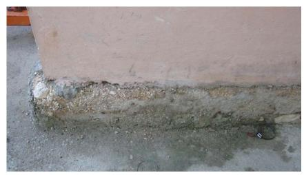
Often the concrete in foundations starts to deteriorate within a few years. This can be caused by the clay in the sand, the lack of Portland cement in the concrete, or a number of other factors. 3 Typical lightly-reinforced framework with masonry infill.
