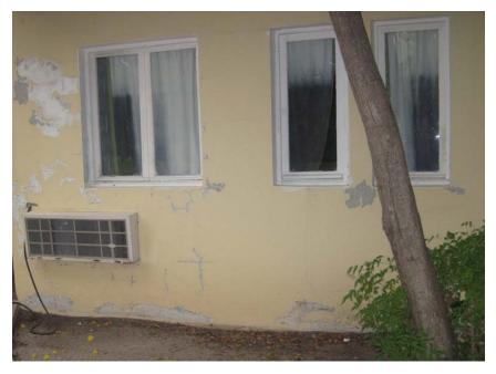
Many of the concrete walls had peeling paint, which indicated that water was coming out of the wall. 11 Many walls had strong angle cracks.
