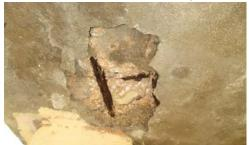
The water table around Jubilee is high, and the water is high in chlorides. Often salt crystals can be seen on the surface of the ground as the soil dries out. Chlorides cause steel rebar to corrode and expand. This causes concrete to crack, which allows more water to enter and corrode more rebar. This photo shows the underside of a water tank which Herb was asked to patch. There was a minor crack
